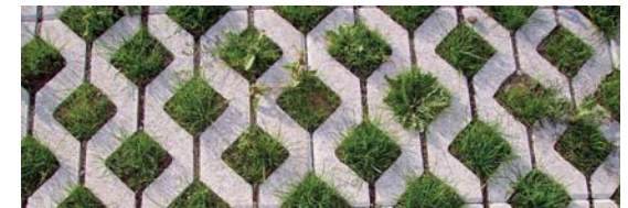
Pervious Driveway Ground Cover
